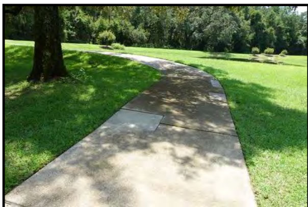
Figure 1 – Previous Repairs
