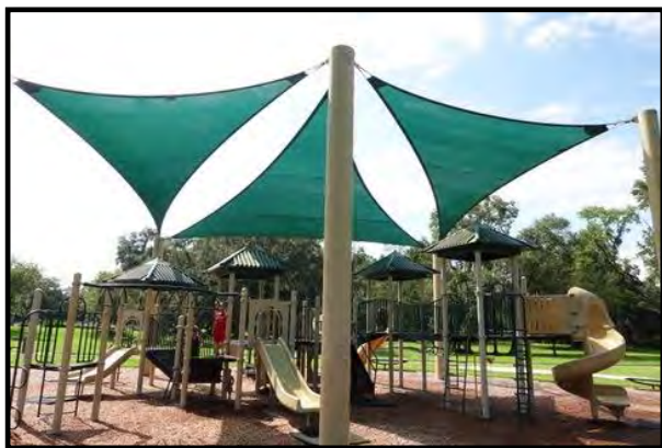
Figure 1 – Playground and Shade Structure
